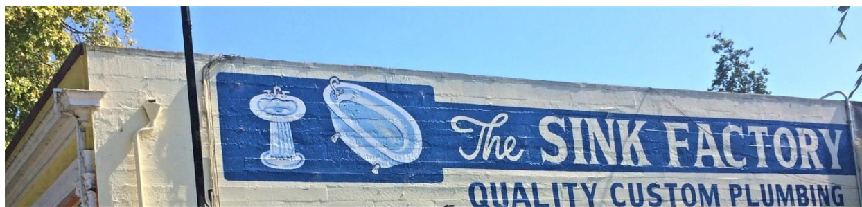
North side of Borg Building, Fran Cappelletti, July 2020
